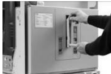
Fig. 5-2: Pull out the handle with two hands
