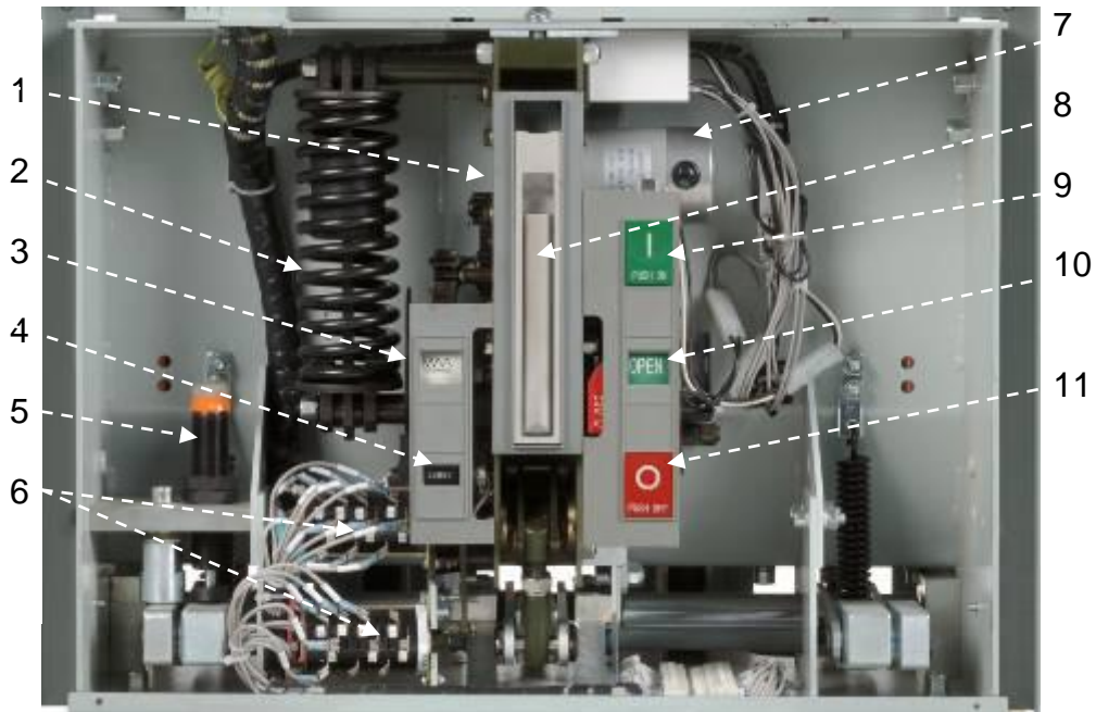
Fig. 3-4: Internal view of W-VACi Circuit Breaker Element
