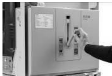
Fig. 5-1: Pull the round handle down
