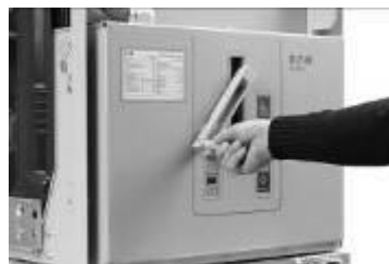
Fig. 5-3: Turn the handle clockwise
