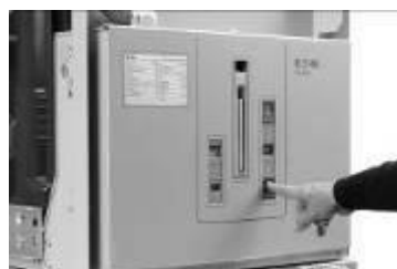
Fig. 5-5: Open manually
