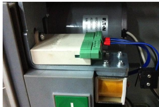
Fig. 5-12B: Mechanism Electromagnetic Interlock
