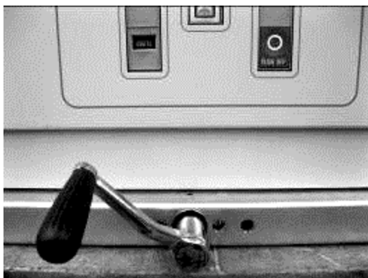
Fig. 5-8: Inserted racking Handle
